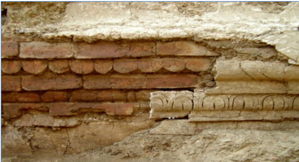
Figure 5: Stucco coating on ornamented brick walls, eastern boundary, Moghalmari
