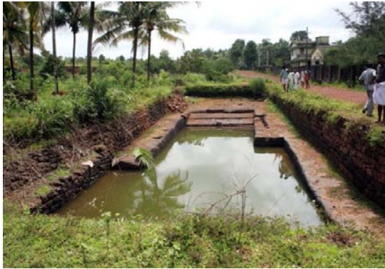
Figure 18: General View of Pond, Ettukudukka
