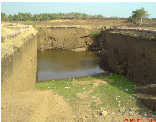
Figure 20: General View of Pond, Mayid
