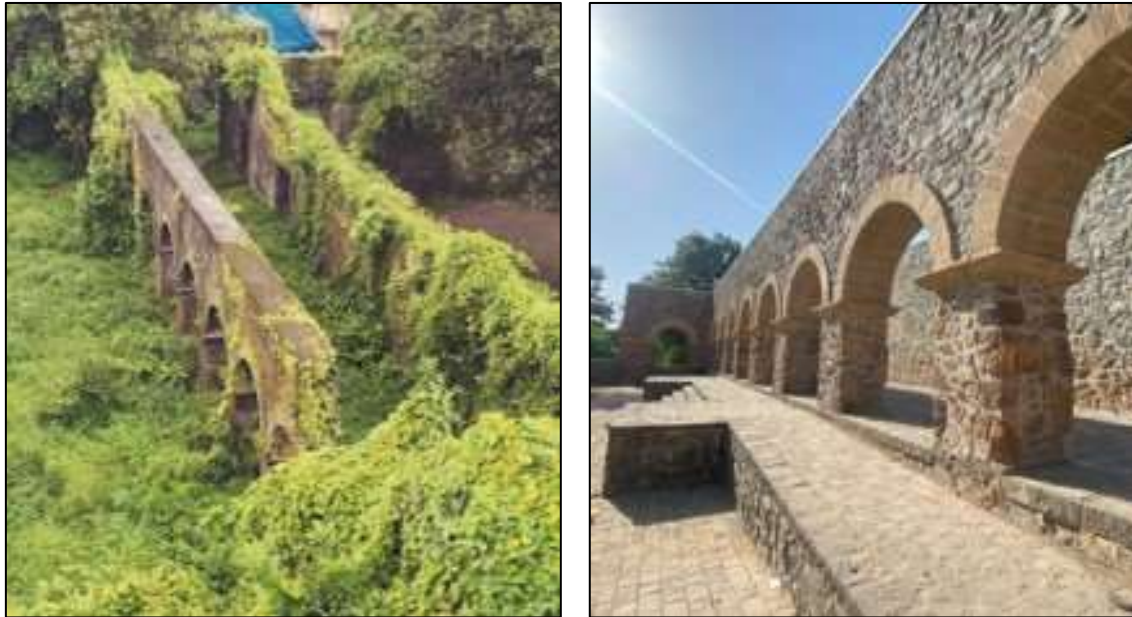
Figure 10a-b: 10a Before and 10b after restoration works at the Ghodbunder fort (© Oke 2024)
