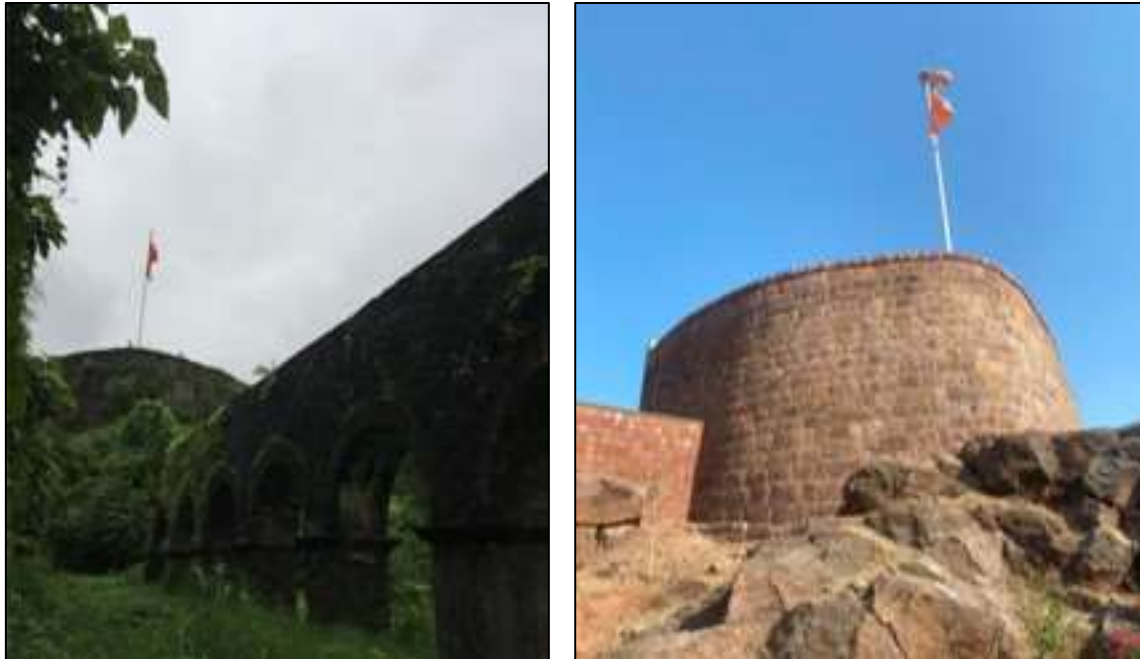
Figure 9a-b: 9a Before and 9b after restoration works at the Ghodbunder fort (© Oke 2024)
