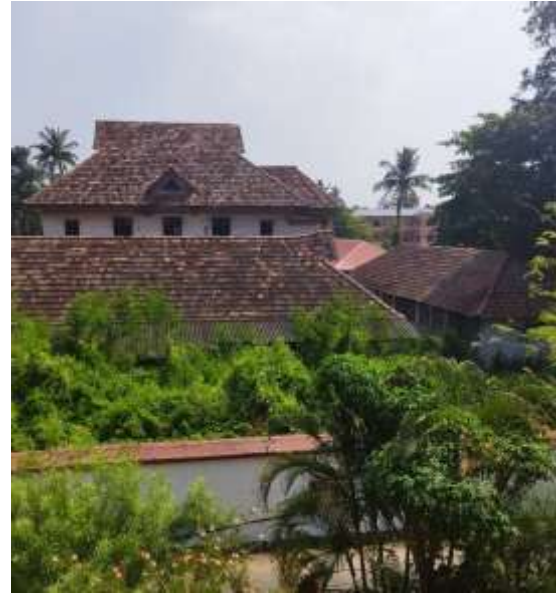
Figure 4: Sprawling Complex once part of Vadassery Amma Veedu
