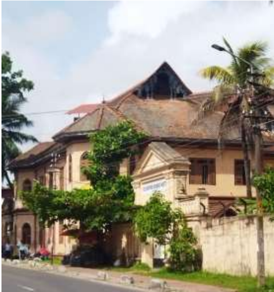
Figure 3: A roadside view of Vadassery Amma Veedu
