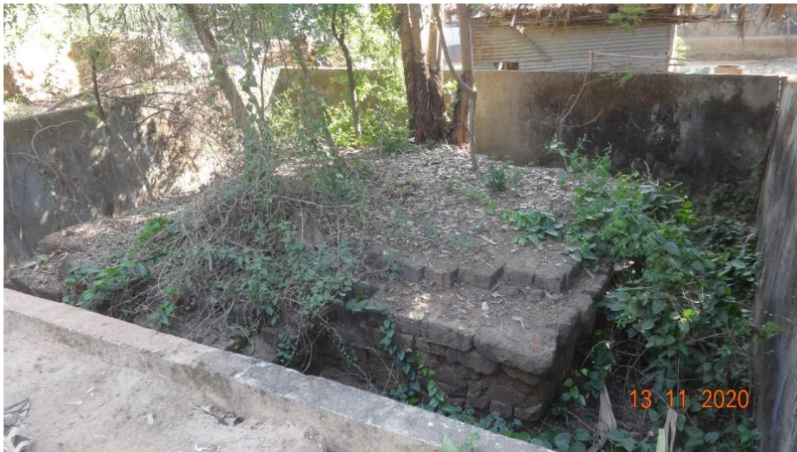
Figure 8: The laterite block structure's base
