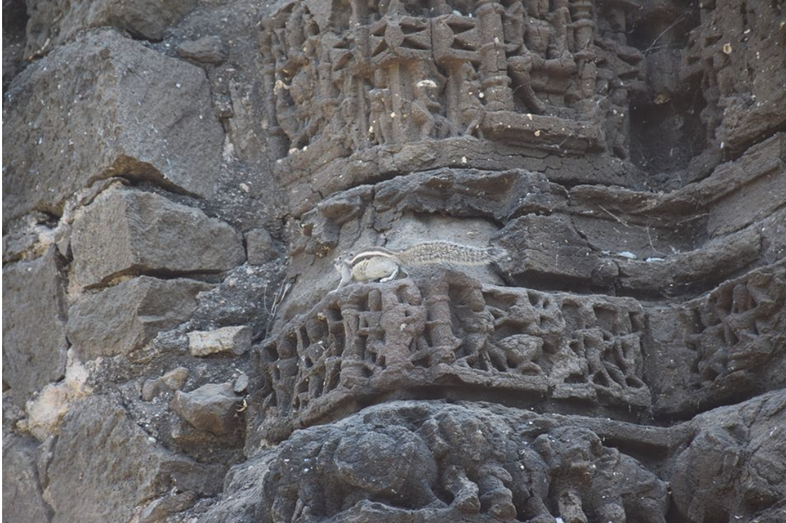
Figure 5: Plinth of Lakshmi Narayan temple, Methi, Dhule (Courtesy: Amar Reddy)
