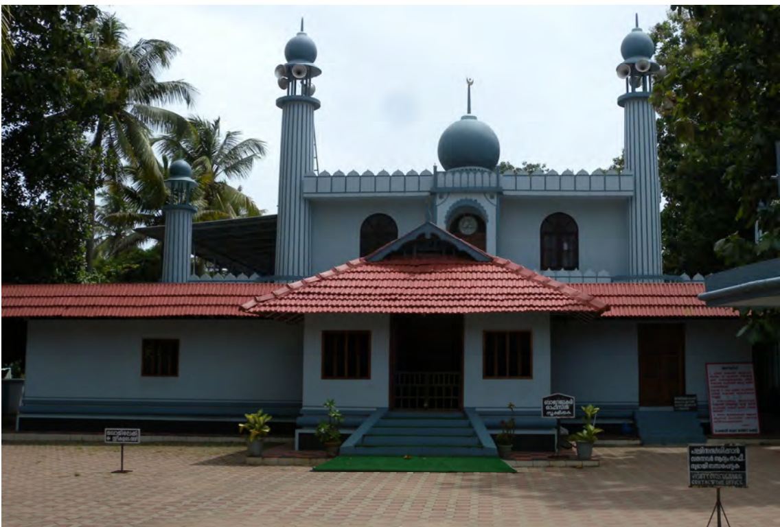
Figure 2: Renovated Cheraman Juma Masjid in Kodungallur
